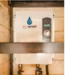
TANKLESS ELECTRIC WATER HEATER
