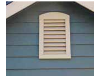
LARGE GABLE VENT
