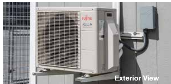
Mini Split Heater/AC Unit 12,000 BTU Unit Requires 110-V A-C 24,000 BTU Unit Requires 220-V A-C Low Temp Units Available for Colder Climates
