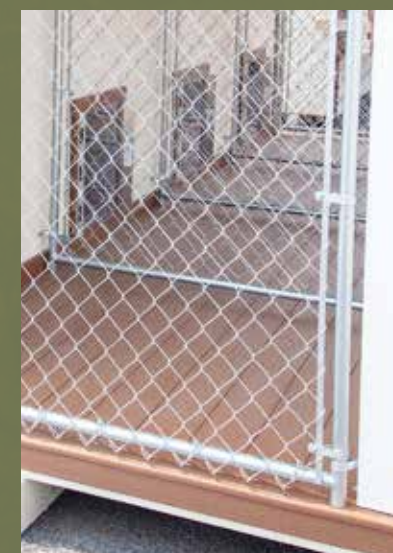
Composite Decking on Runs
