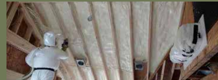
SPRAY FOAM INSULATED FLOOR
