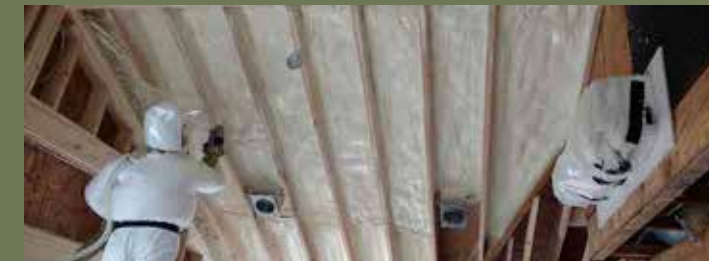
SPRAY FOAM INSULATED FLOOR
