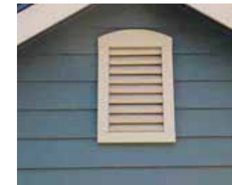
LARGE GABLE VENT
