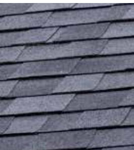
Shingle Roof 30 - Year Architect Shingles
