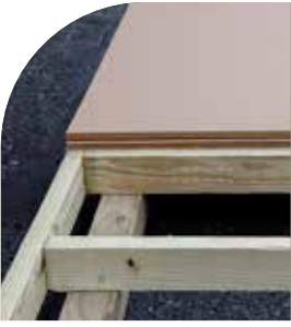
Pressure Treated 2" x 4" Floor Joists and 4" x 6" Runners
