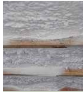
R-13 Closed Cell Spray Foam Insulation In Floor
