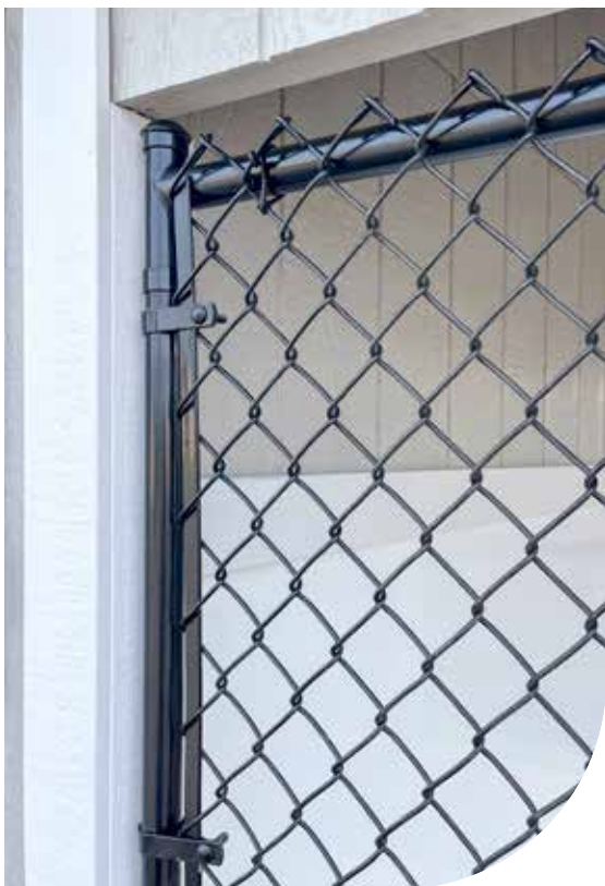
Upgraded Vinyl Coated Chain-Link Fencing
